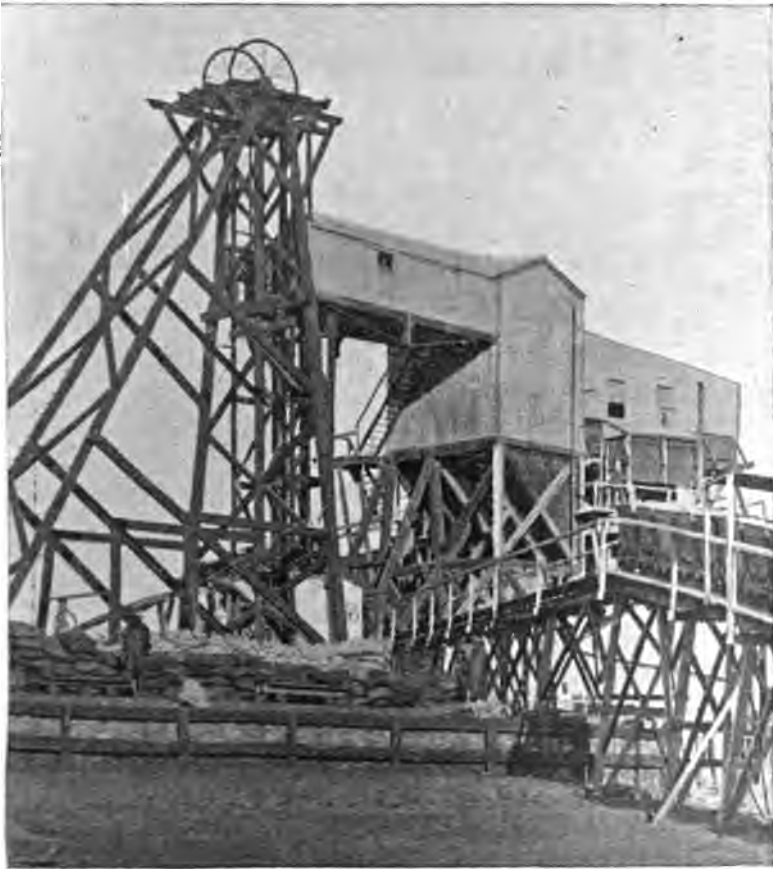
FIG. 4.—HEAD-GEAR AND BINS.
